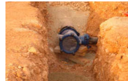
Pipeline trench filling
